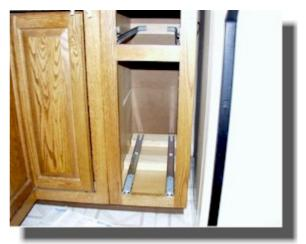
**Step 2**. Measure width of cabinet opening. Make your trash box at least 1/2" **smaller** in width than this measurement. Depth will be approximately 16", and height from bottom of cabinet approximately 18". Fasten together with 1 1/2"-2" finish nails. We used wood shelving material from Lowe's that is 3/4" thick, white plastic coated particle board. The plastic coating makes for easy cleanup, and a finished product as soon as your done assembling it.
